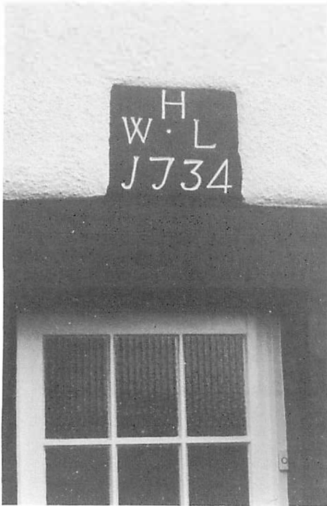
(a) Lintel, Eamont Bridge
