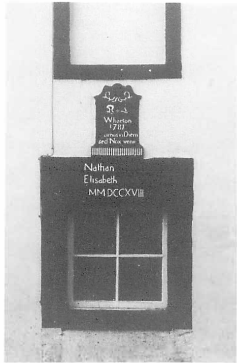
(b) Lintel, Eamont Bridge
