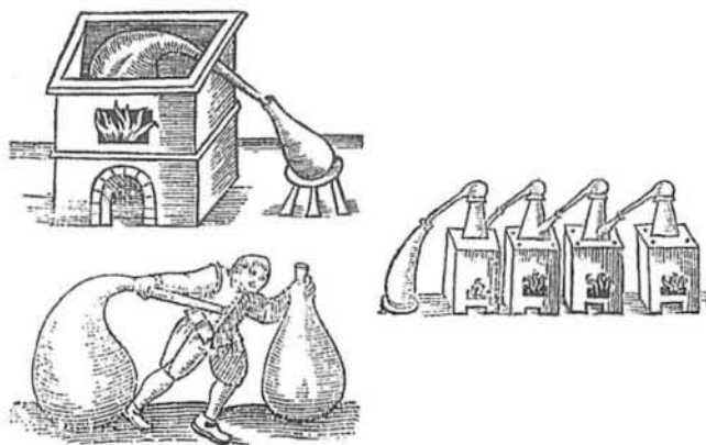
Fig. 10: Left: retorts, and right: cascaded stills, from French's Art of Distillation 1667 pp78, 31.
